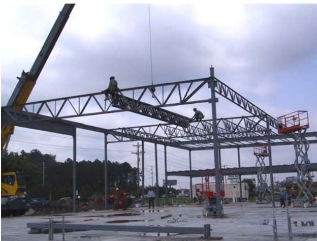
Figure 14 Bundle of shortspan joists being placed at mid-span of Joist Girders
