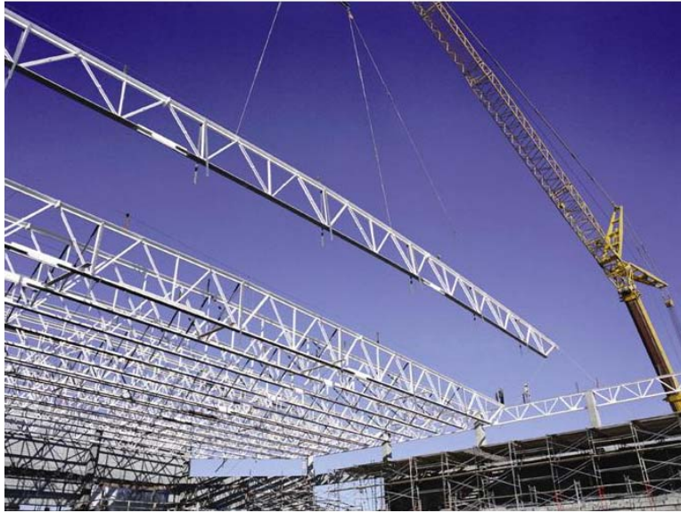
Figure 18 Longspan joist with bolted splices at two locations being erected
