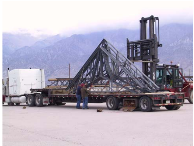
Figure 3 Non-standard SJI Product – Scissor Joist
